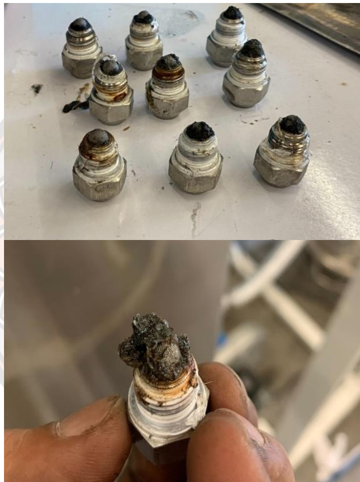
Figure 34 Figure 35 The packed bed material clogs the spray heads.
