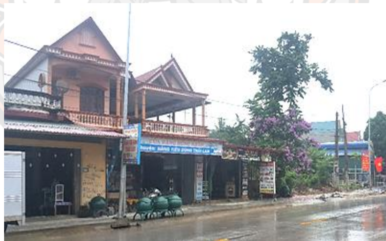
Figure 57: Hybrid architecture in house construction of VKHH in Làng Thái Lan
