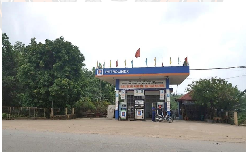
Figure 23: VKHH's petrol station
