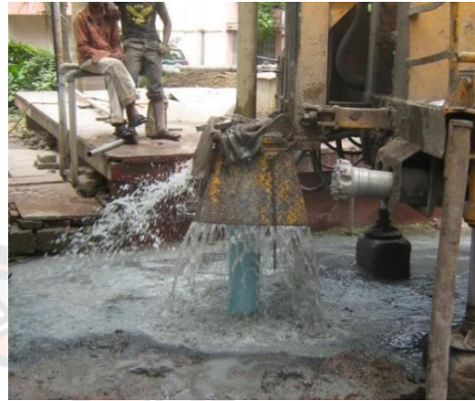
Figure 21 Borewell being drilled to tap a deep aquifer
