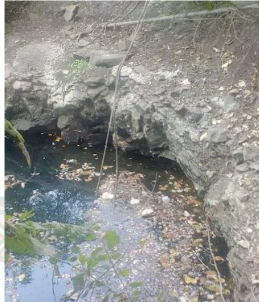
Figure 19 Formation of a water pool by water seepage through jointed flows
