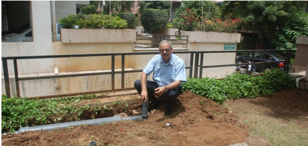
Figure 28 Installed PVC barrel-based sand filter
