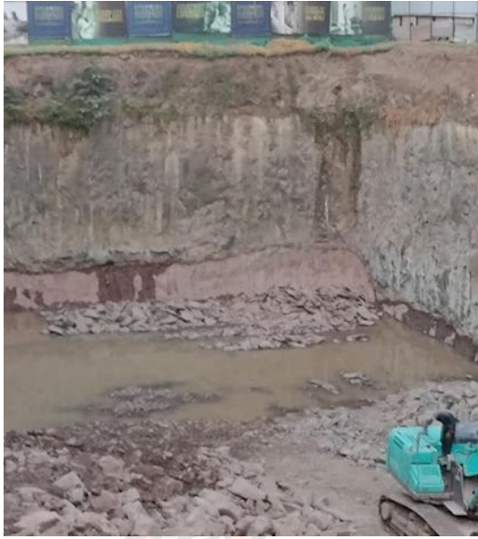
Figure 18 Water seepage along the flow unit contacts
