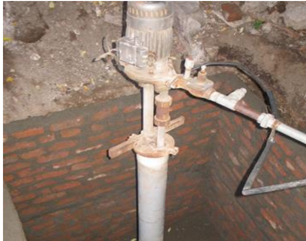
Figure 26 Bare pit with brick lining for recharge purposes
