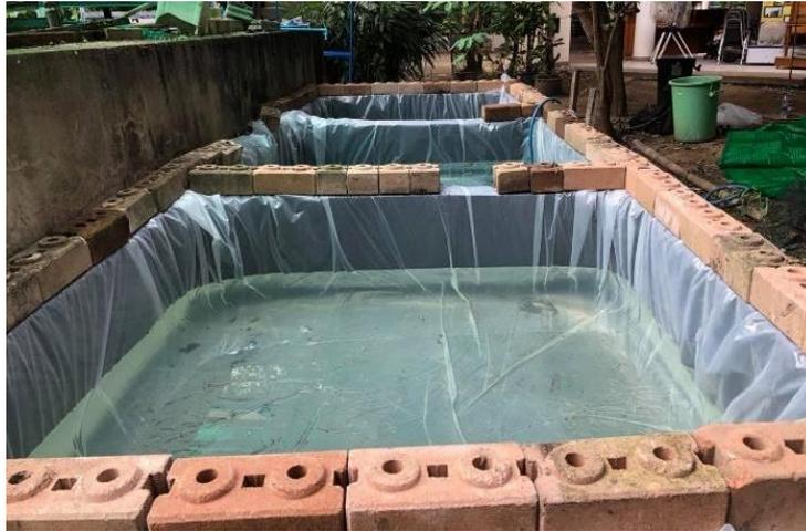
**Figure 37** The fishponds were built by using interlocking bricks with 2 m of width, 2 m of length and 70 cm of height
