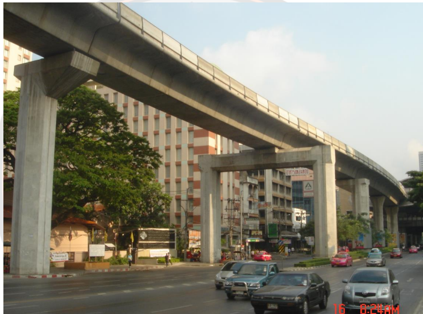
Figure 1 Box girder bridge for BTS sky train in Bangkok, Thailand.
