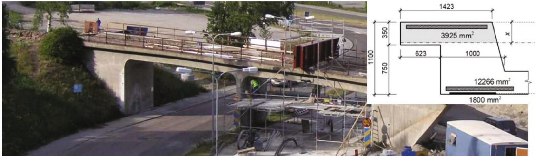
Figure 47 The tested railway bridge [36]
