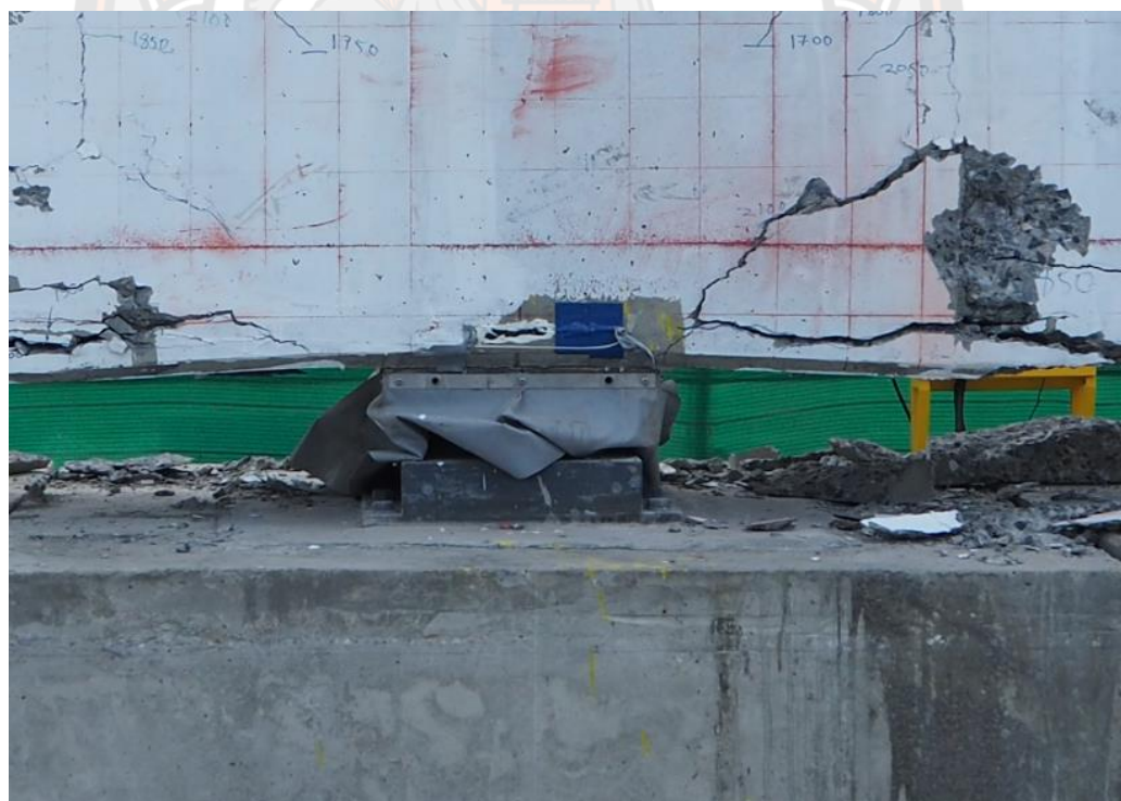
Figure 161 Bearing B-02 after test
