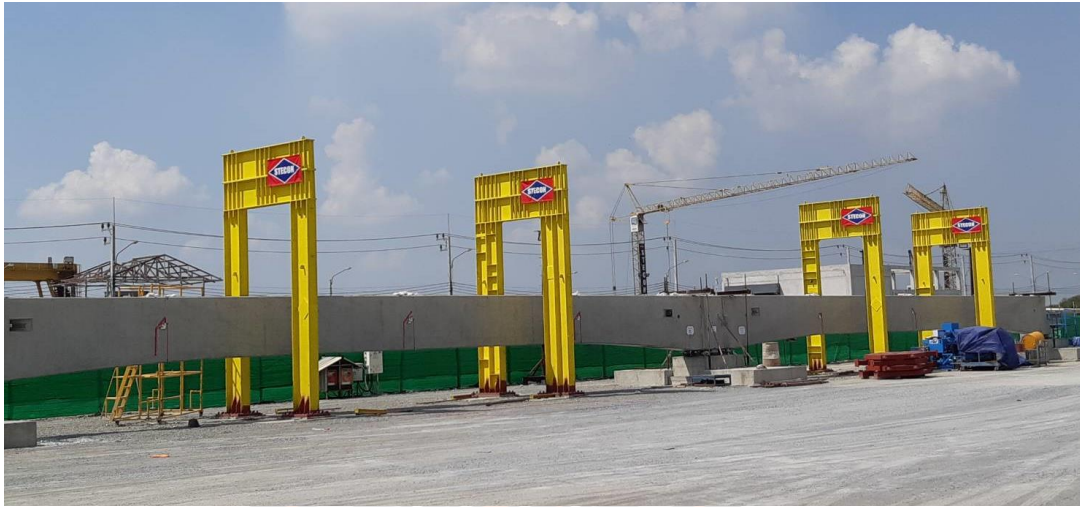
Figure 88 Typical view of the FPPC monorail bridge girder.
