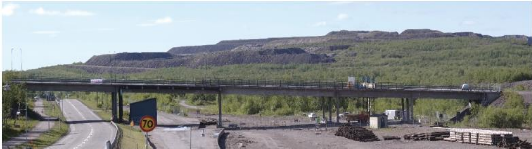
Figure 48 Photograph of the Kiruna bridge, view from north [36]
