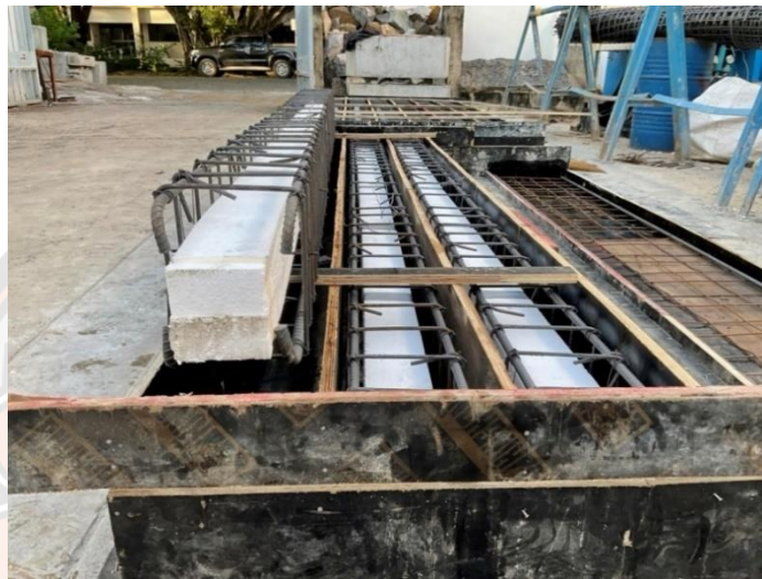
Figure 106 Installation of foam in steel bars
