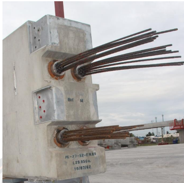
Figure 83 Typical post-tensioning of the FPPC girder.
