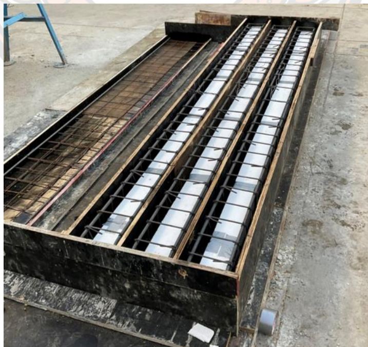
Figure 107 Installation of steel bars in formwork
