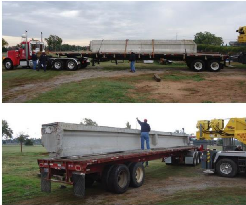
Figure 30 Arrival of girders at Fears Lab on flatbed trailers on October 8, 2013 [34]
