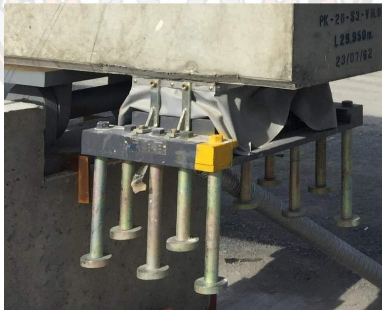
Figure 157 Typical view of bearing.
