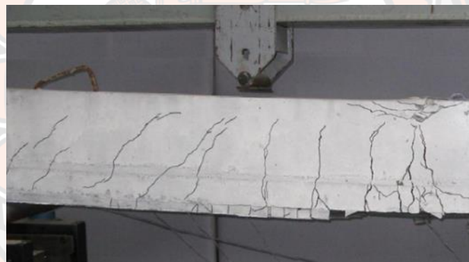
Figure 61 Typical failure mode of RC beam [39]
