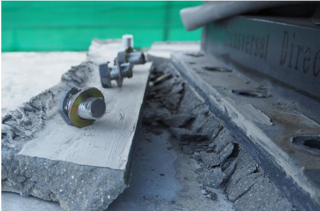
Figure 162 Ultimate failure of bearing B-01.
