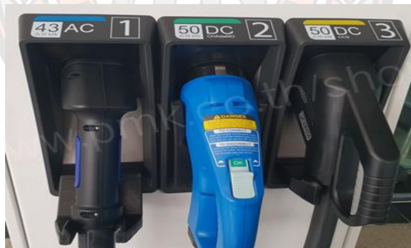
FIGURE 5 NORMAL CHARGER AC TYPE2 AND QUICK CHARGER DC CHADEMO, CCS TYPE2
